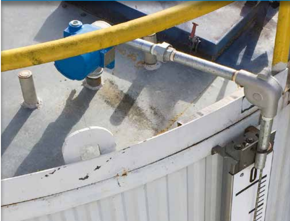
Photos represent typical installation of the MCG 2420 Transmitter and 92302 Liquid Level Indicator and are not from the Puerto Rico power plant.
