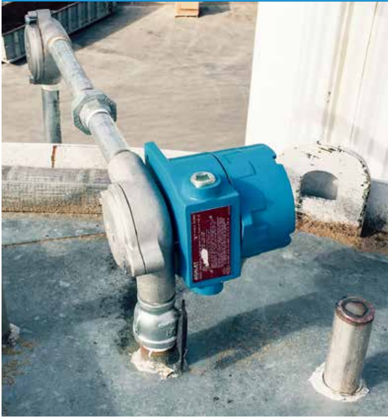
Photos represent typical installation of the MCG 2420 Transmitter and 92302 Liquid Level Indicator and are not from the Puerto Rico power plant.
