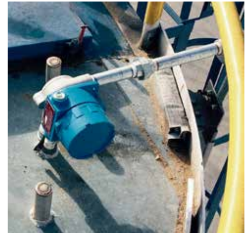
Photos represent typical installation of the MCG 2420 Transmitter and 92302 Liquid Level Indicator and are not from the Puerto Rico power plant.
