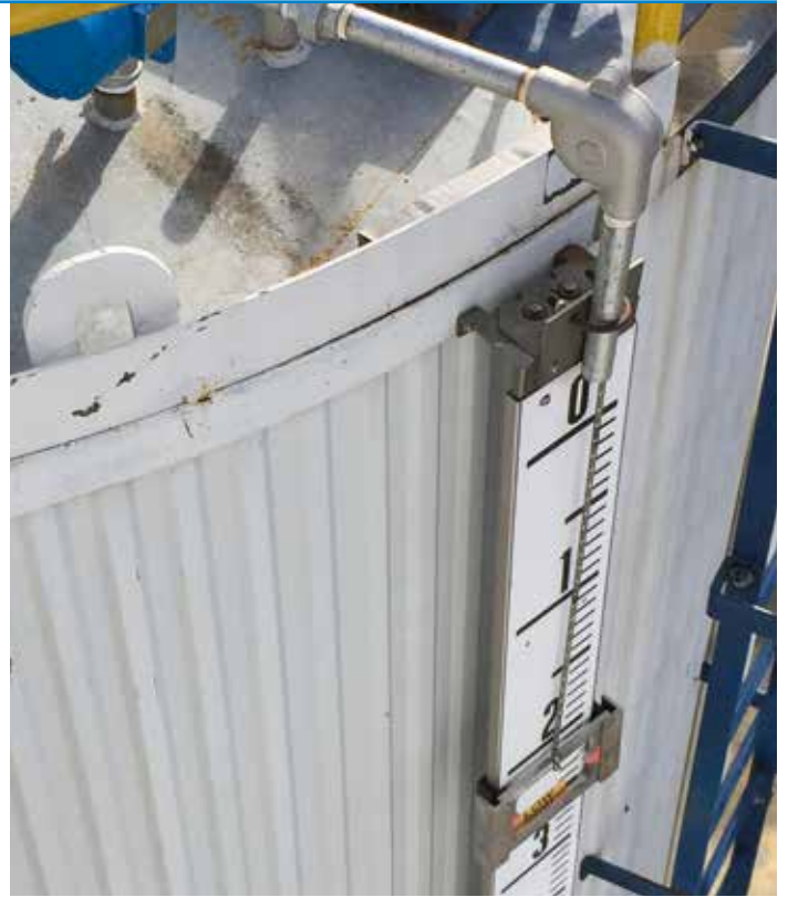
Photos represent typical installation of the MCG 2420 Transmitter and 92302 Liquid Level Indicator and are not from the Puerto Rico power plant.
