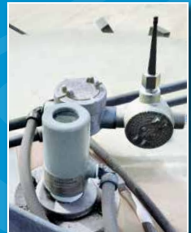
evo 2600 Radar Gauge Wireless Installation
