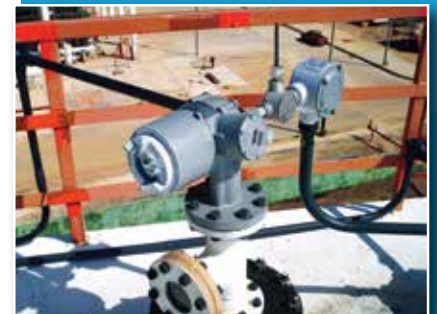
MCG 1500SFI Smart Flash Infrared Servo Gauge Wireless Installation
