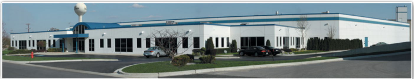
World Headquarters in Hillside, IL
